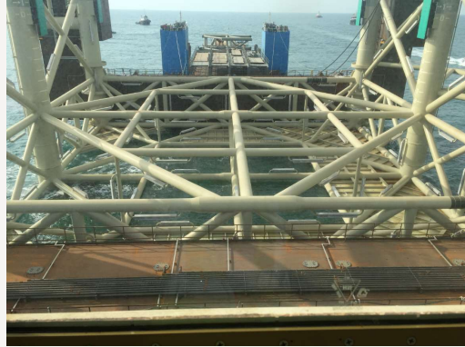
Ballasting on WishWay
