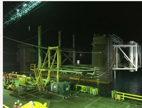
JKT before ballasting
