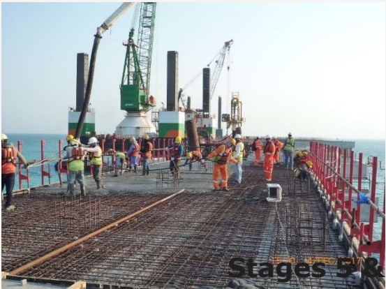
Stages 3 & 4 in-situ concreting
