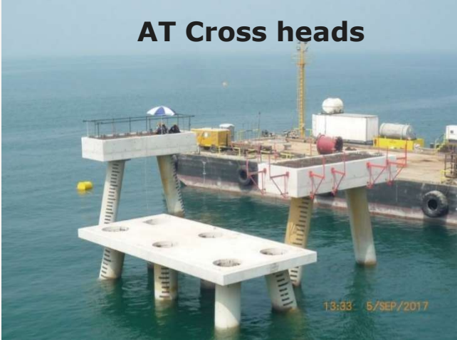
Stages 1 & 2 in-situ concreting
