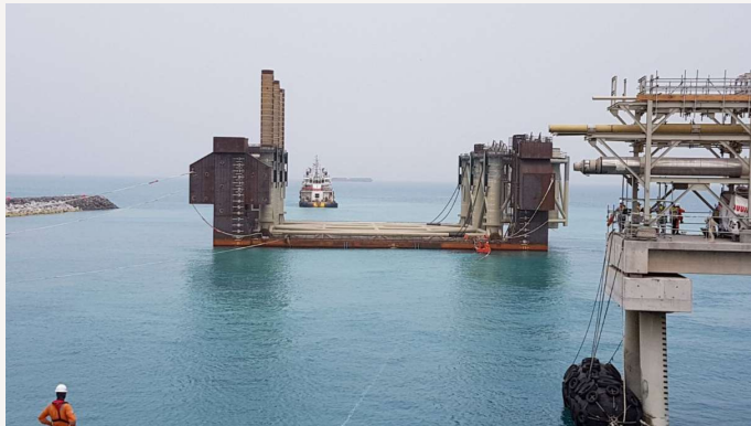
JKT pulling from HD-1000 to its designated position
