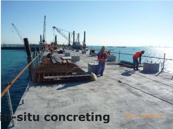
Stages 3 & 4 in-situ concreting
